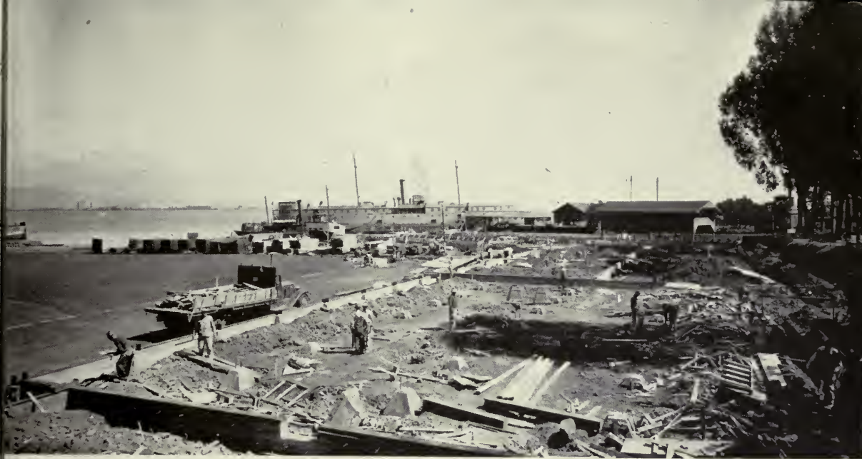
New Construction on Filled-in Land, Yerba Buena Island •
